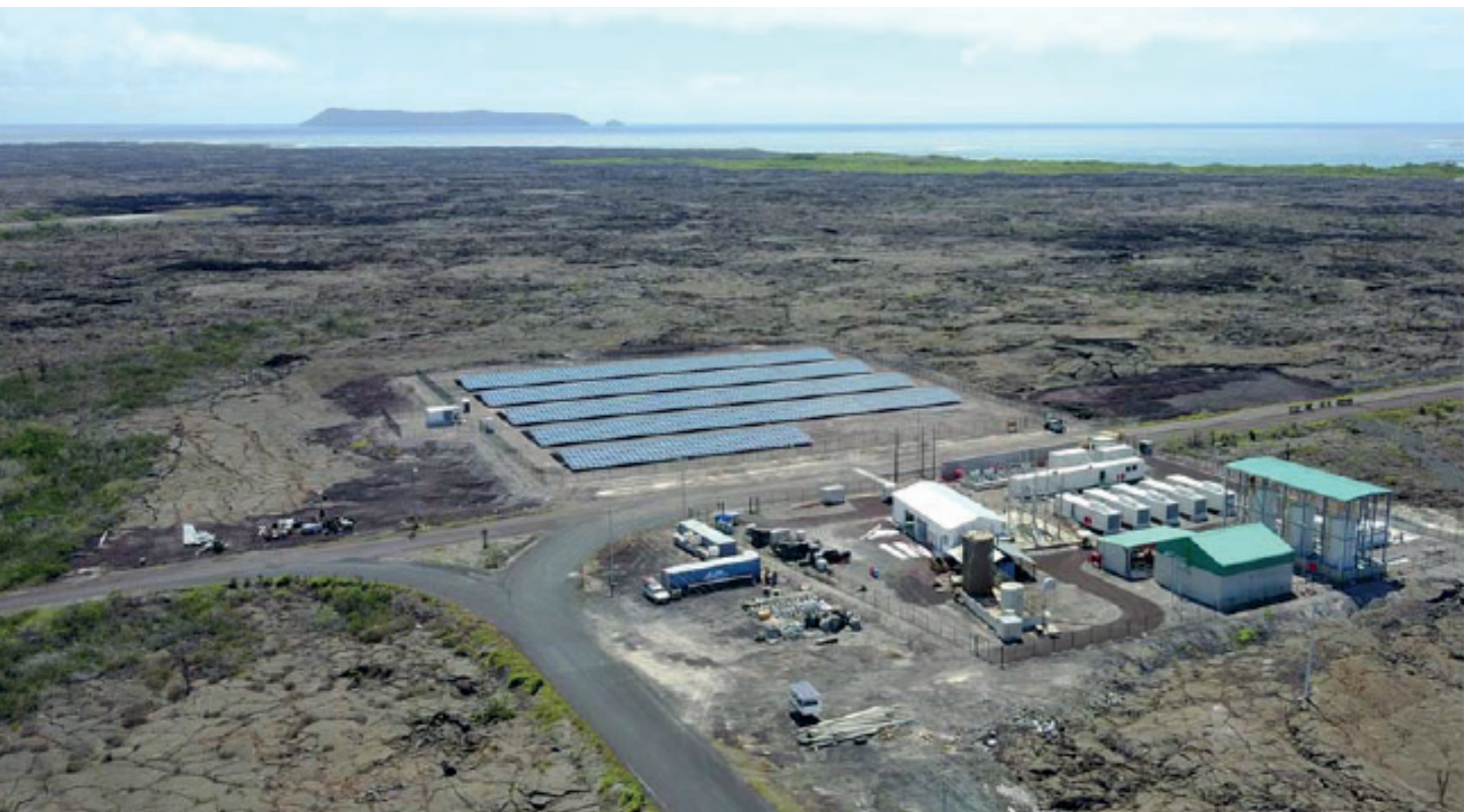
100% Renewable Energy Hybrid Power Plant on Galapagos Island Isabela. Built from Siemens AG and Designed from VWP
